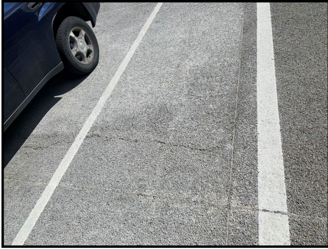
Linear Cracks
